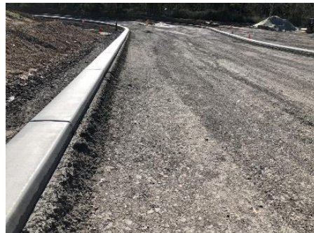
Image 2: Kerb and gutter concrete incorporating Shoalhaven RCG glass
